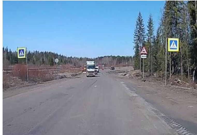
Figure 4: Marking for pedestrian crossing is absent
