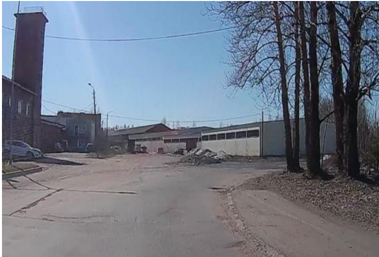
Figure 3: Abrupt ending of sidewalk
